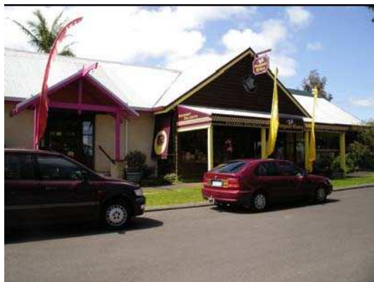
Single storey retail/tourist outlet, located on Bottrill Street. Constructed of rammed earth and timber panelling, with a pitched zinalume roof. Building is approx. 20 to 30 years old.
