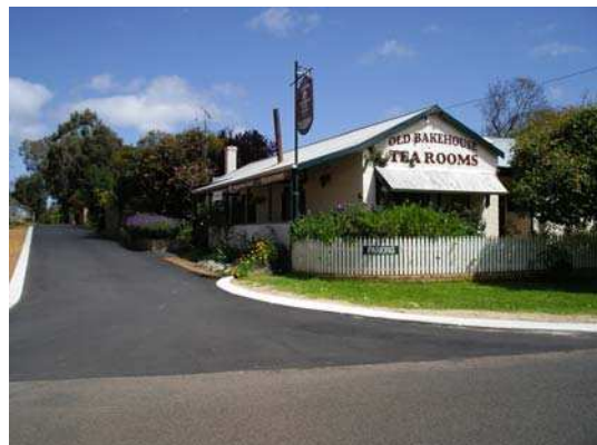
Single storey tearooms on O'Brien Street. Circa 1940s Group Settlement building of asbestos/fibro and pitched zinalume roof. The building is set in attractive gardens with a bordering picket fence.
