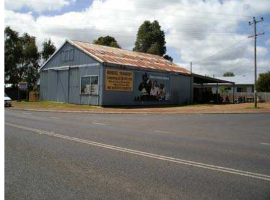
Single storey machinery and truck stop shed located on Bussell Highway corner Waverley Street. Walls and roof of corrugated iron. Circa 1951.
