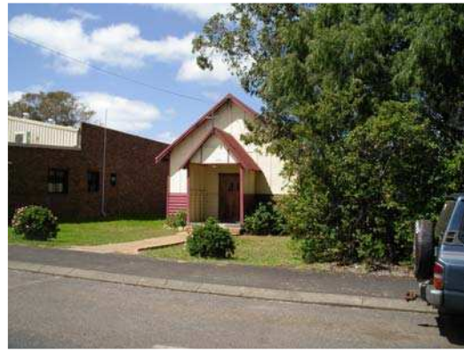
Original Congregational Church, opened 1928. Walls of weatherboards and asbestos/fibro, roof is red corrugated iron. Located on Bussell Highway in the town centre, and set back from the footpath with a "green" forecourt.
