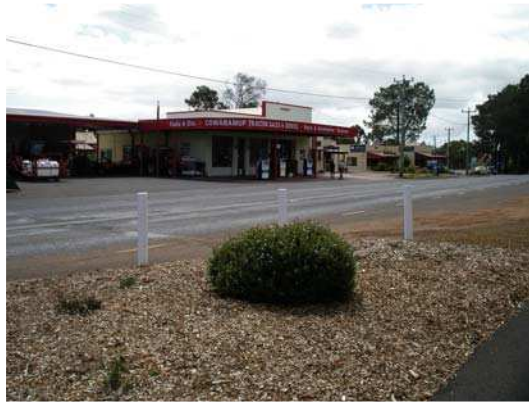
Single storey garage with a flat corrugated iron roof and walls of painted brick and weatherboard. Circa 1940s.
