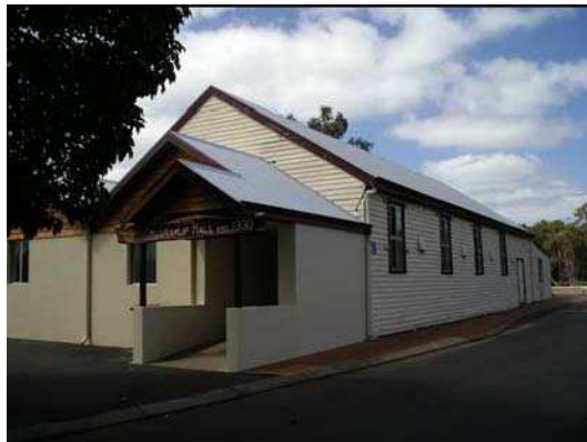
Cowaramup Hall, built 1930 and enlarged and somewhat modernised since. Walls of weatherboard and rendered brick, roof is zincalume and colorbond. Located on the corner of Bussell Highway and Hall Road, set well back from the Highway.
