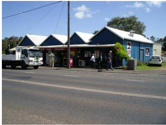
Single storey building circa 1923. Walls of weatherboard and asbestos/fibro, a pitched roof of zinalume with four gables facing the street. Centrally located on Bussell Highway it is one of the most visually prominent buildings in town, with its striking roof form and brightly painted walls.
