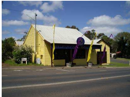
Older style circa 1940s Group Settlement Scheme building located on the corner of Bussell Highway and Bottrill Street. Walls of painted weatherboard with a steeply pitched zinalume roof.
