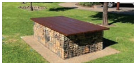
Gabion walls with timber slatted top
