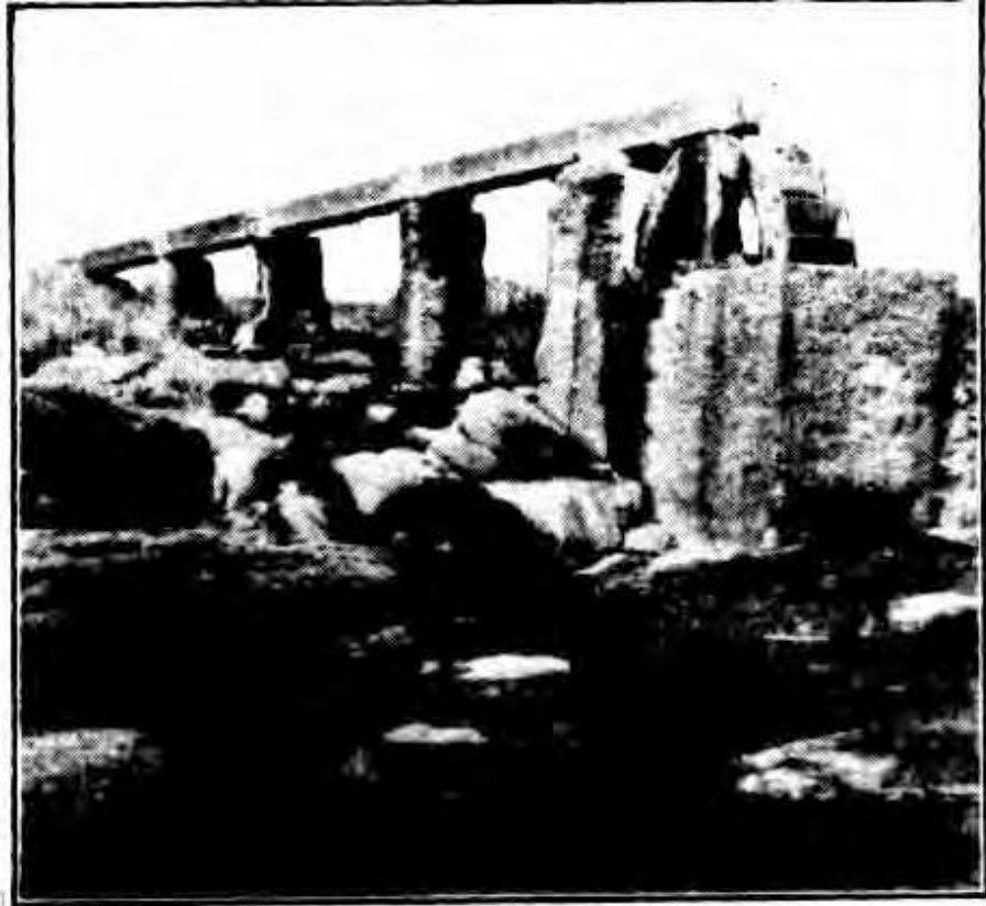
The quaint old water-wheel, driven by water from a swamp, which conveys water to the quarters of the keeper of the Cape Leeuwin Lighthouse, in Western Australia
