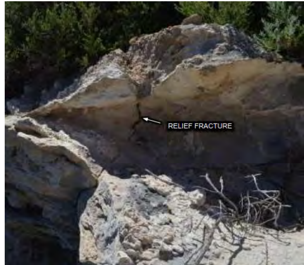
Fracture from Golder 2017 inspection
