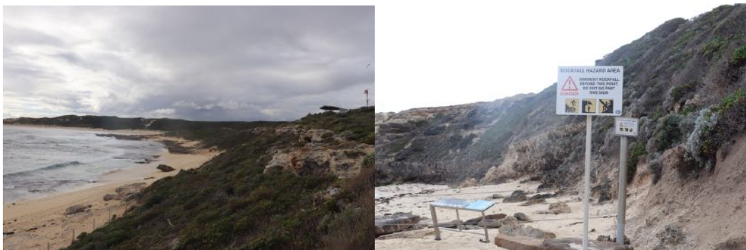
Limestone coast at Main Break (left) and Riffle Butts (right) with rockfall hazard signs.
