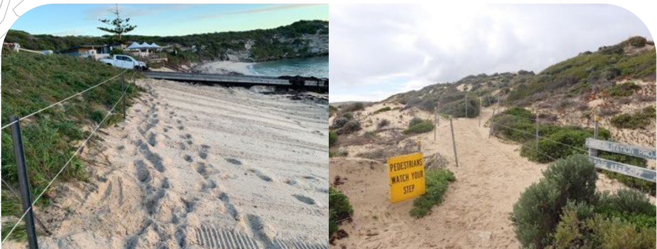
Figure 2.7 - Sand Nourishment at Gnarabup Beach in 2022 (left), and a local path diversion following storm erosion in 2018 (right)
