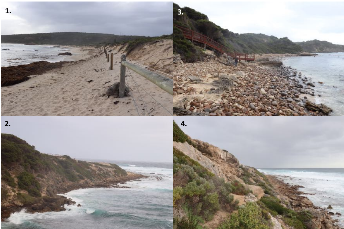
Melaleuca Beach where fencing has been rebuilt in response to foredune erosion (1), exposed cobbles beneath sandy beach and beach access stairs at Huzzas (2), limestone cliffs and beach access stairs at South Point (3, 4)
