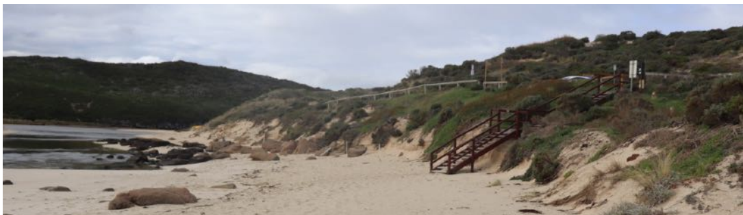
Margaret River entrance, with erosion beneath access stairs to the carpark.
