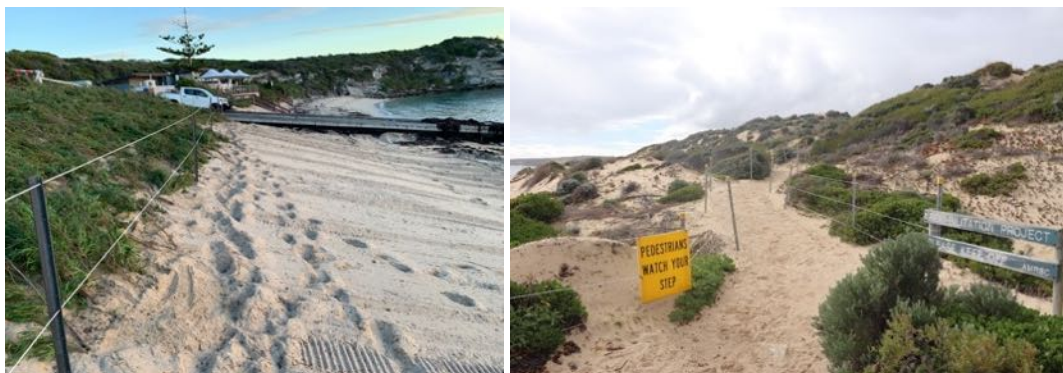
Figure 4-5 Sand Nourishment at Gnarabup Beach in 2022 (left), and a local path diversion following storm erosion in 2018 (right).
