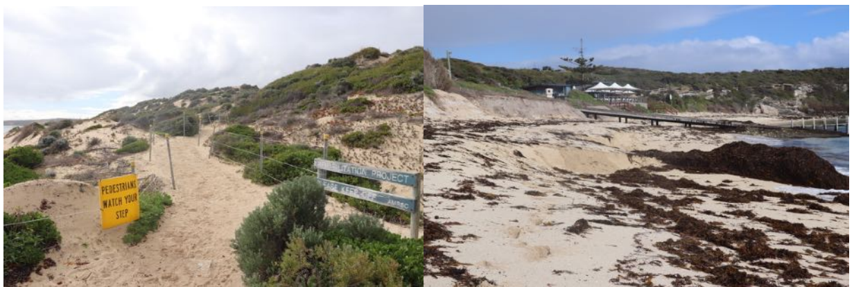
Gnarabup coastal path diversion in response to foredune erosion (left), sand nourishment works and beach response to wrack depositions (right).
