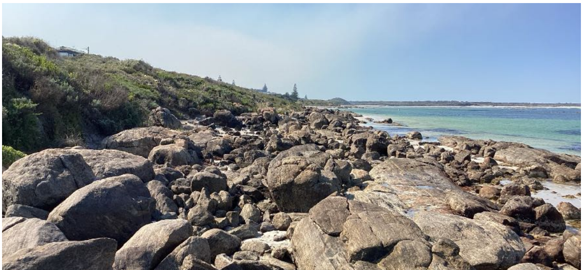
Rocky coast at Albany Terrace. Survey shows rock up to 2.0m AHD but with lower areas backed by sandy foredune have potential for erosion with higher sea level.
