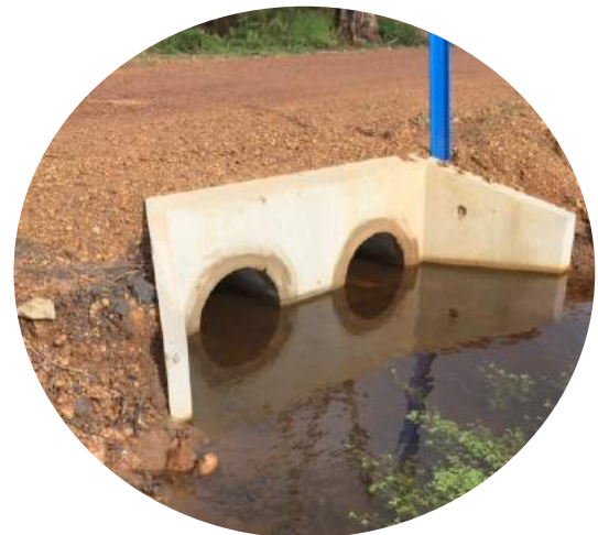
Above: Twin culvert drainage to Bullant Drive (typical project)
