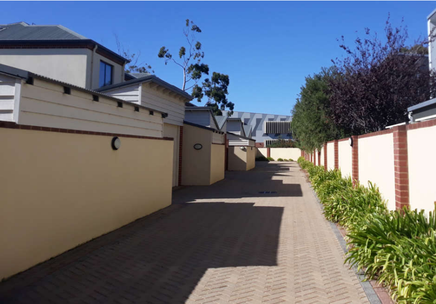
Photo 2: View of common driveway and southern elevations of Grouped Dwelling complex at 15 Station Road
