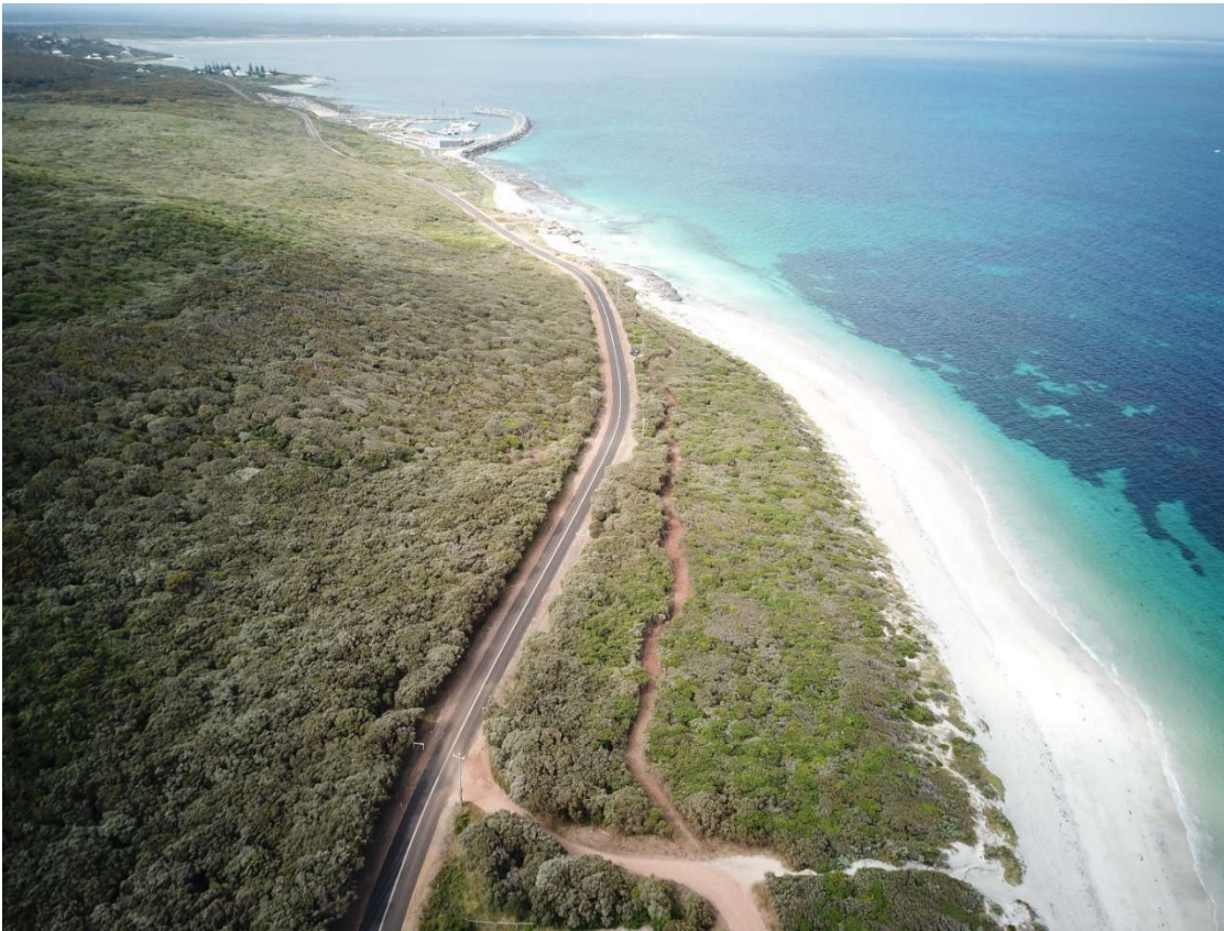
Figure 2 – Aerial View of existing path/Dead Finish Road junction looking east
