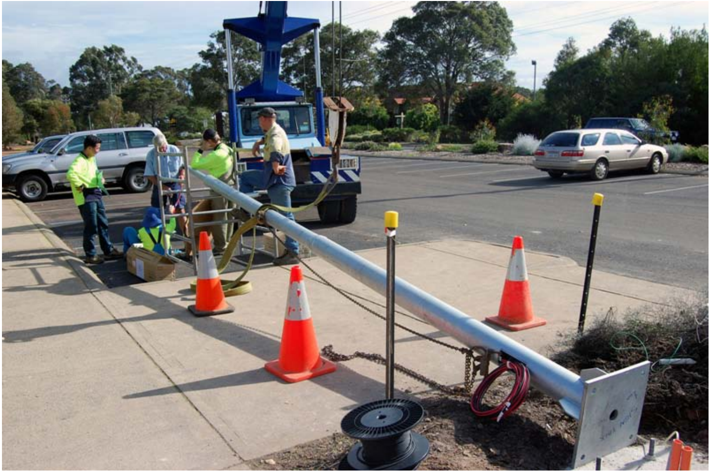
Installation of turbine
