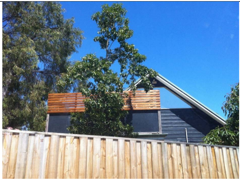
Image: Screening applied to the balcony as viewed from the east.
